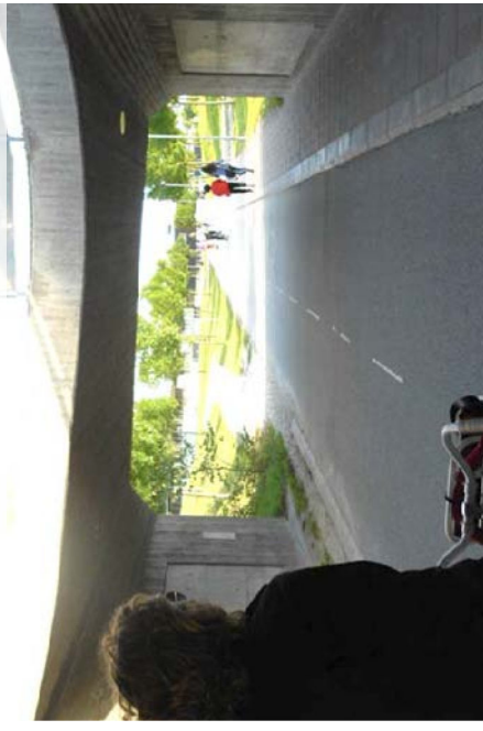
Figure: 10.52 Underbridge (cycle and pedestrian-only) with divided carriageway above to create opening – Lund, Sweden
