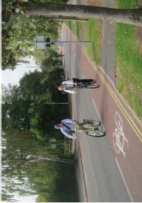
Figure 6.33: Red pigmented asphalt is used for all cycle routes in Cambridgeshire
