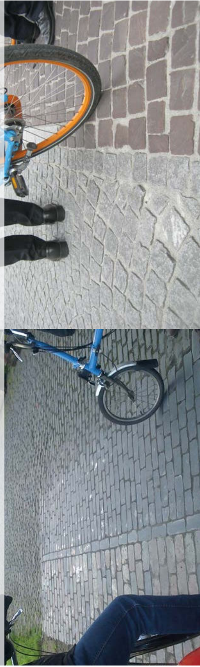
Figure 7.9: Trial site in Bristol to provide smoother surface, and similar application in Bruges with setts in a different colour from the adjacent traffic lane.
