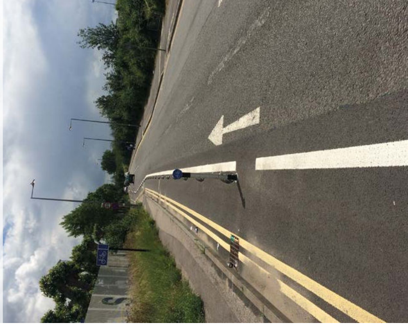
Figure 6.17: Low level light segregation features adjacent to a mandatory cycle lane
