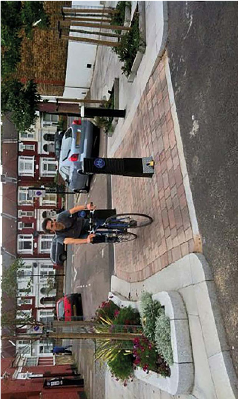
Figure 7.1: Simple modal filters can reduce through traffic while retaining cycle and pedestrian access. The central position enables kerbside car parking to be provided without blocking the facility, and the lockable bollard enables emergency access, Haringey.
