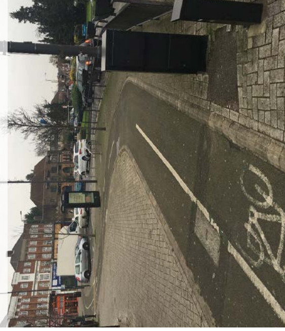
Figure 10.36: Footway-level cycle track around large roundabout, Harrow
