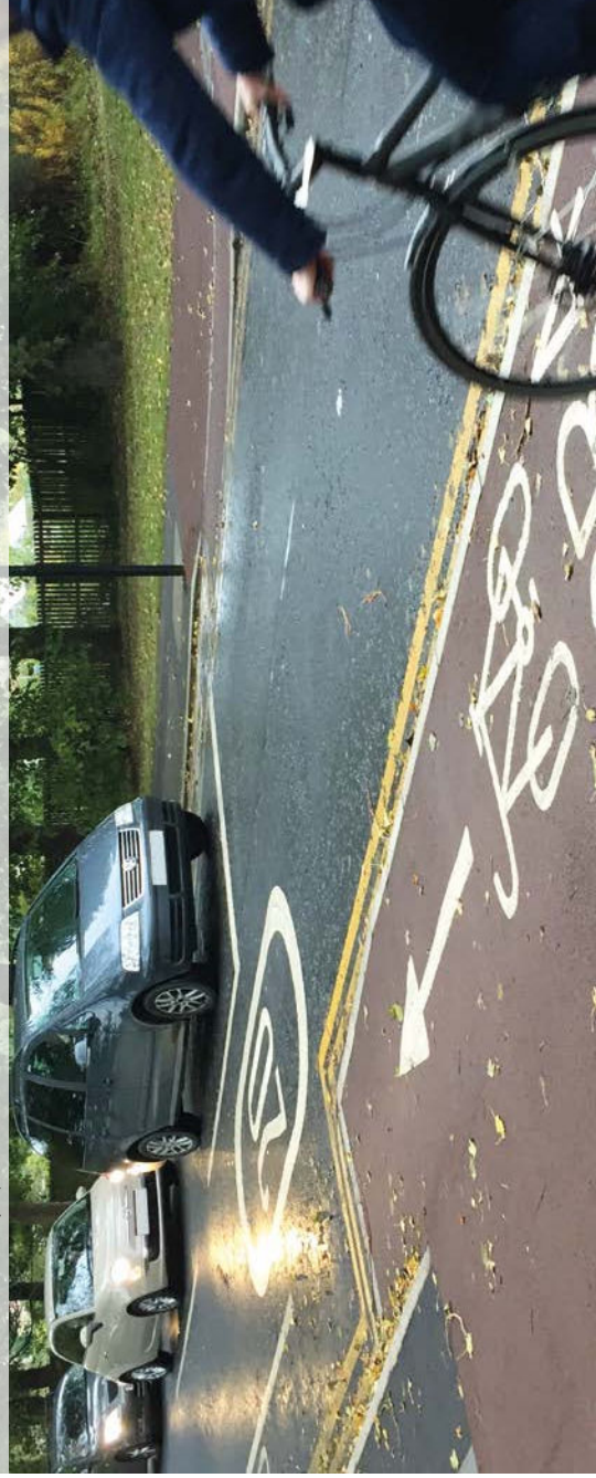
Figure 9.2: Cycle track entry and exit ramps at a signalised junction, Newcastle (Note: double yellow lines not required across transition ramps)
