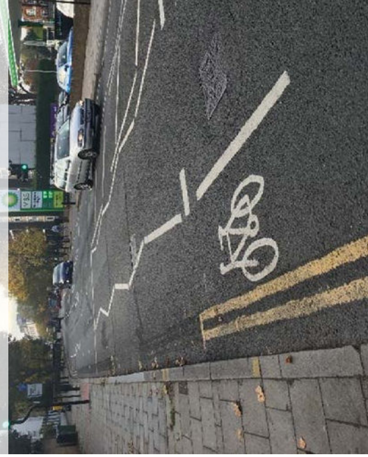
Figure 6.19: Zig-zag markings placed away from the kerb to continue cycle lane, Greenwich
