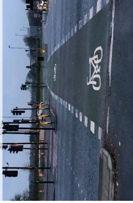
Figure 10.9: Single-stage straight-over cycle crossing next to multi-stage staggered pedestrian crossing, South Gloucestershire
