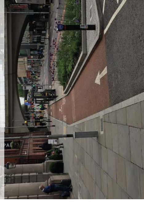
Figure 9.4: Cycle lane to cycle track transition
